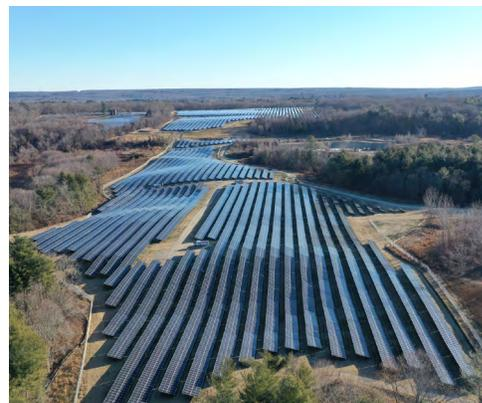
Using racking technology like the **GLIDE fixed system**, designed with reduced hardware and parts, helped to speed things up. Inherently adjustable with a wide range of front-edge heights, GLIDE installation is 33% more efficient than other fixed systems while allowing for more snow clearance and less drift.
