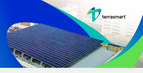
Building a solar canopy on top of a parking garage is an effective way to increase the presence of renewable energy systems in urban environments. Beyond the benefit of solar, canopies also provide shading for vehicles parked on the top level of the garage. Canopy structures are designed to be minimally invasive, meaning existing parking spaces will not be impacted in any way.
