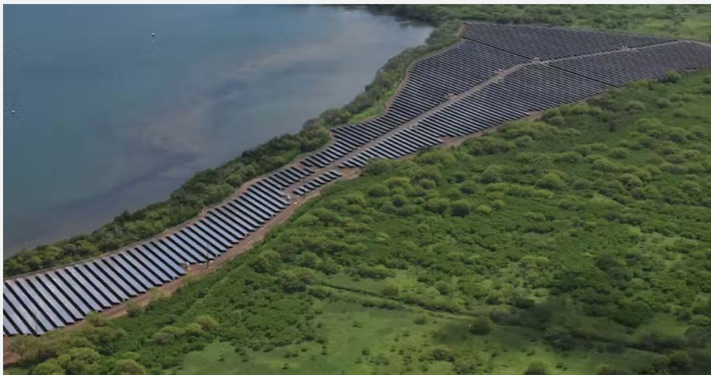
Waipio Solar PV Station on Oahu
