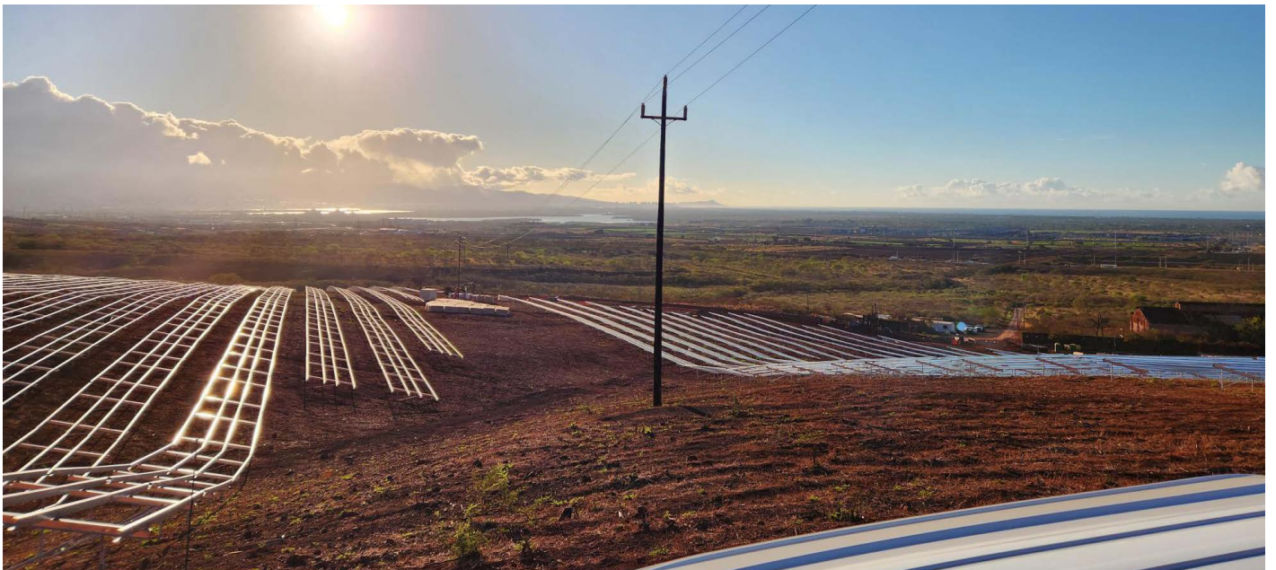
18-MW solar system in West Oahu
