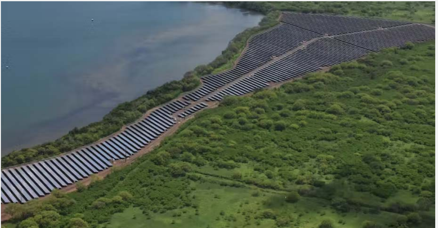
Waipio Solar PV Station on Oahu
