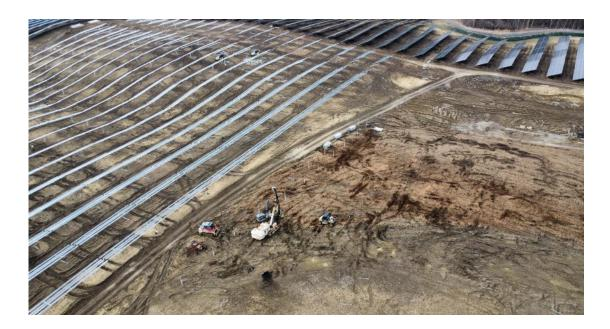
"If we are delayed with our racking install, it's a disaster for the project. It doesn't matter how many test pits you do, there's always the unknown," Hill explains. "We've done countless geotechnical tests on a job when—all of a sudden—we hit a ledge and now we're stopping. Using ground screws wipes out refusals and locks in our schedule."
