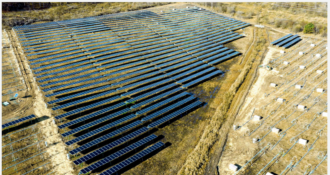
PureSky’s Green Dale site under construction
